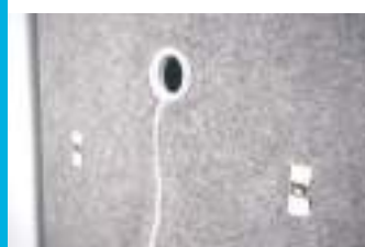
PRE CUT HOLE FOR CABLE MANAGEMENT
